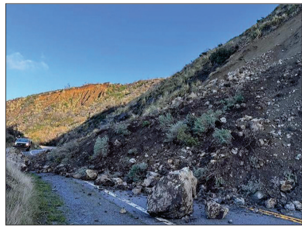
PHOTOS/WEATHERTECH RACEWAY (LEFT), CALTRANS (ABOVE)
