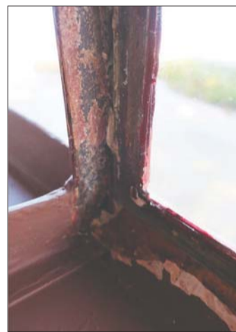
The Frank Lloyd Wright house (above) at the south end of Carmel Beach suffers the effects of constant exposure to the ocean, including rusted and corroded windows (right).
