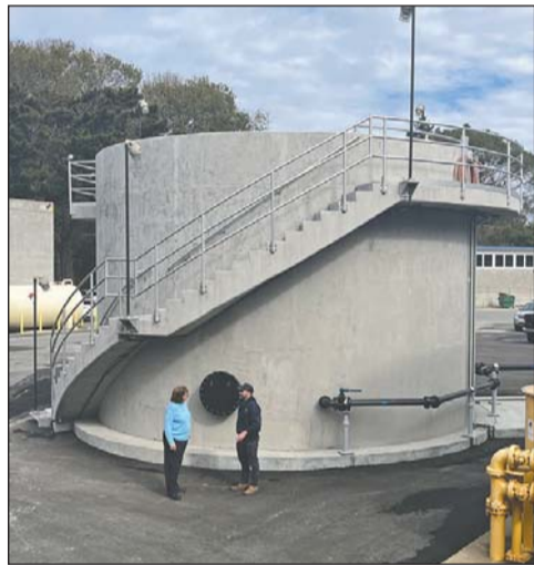
A major upgrade at the CAWD sewer plant included installing a second digester (left), which breaks down organic waste. The work also included replacing all the plant's motor control centers, which plant engineer Patrick Treaynor (right) shows the Pine Cone.
