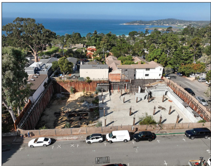
DRONE PHOTO/MIKE BUFFO, HOUSE OF 8 MEDIA
