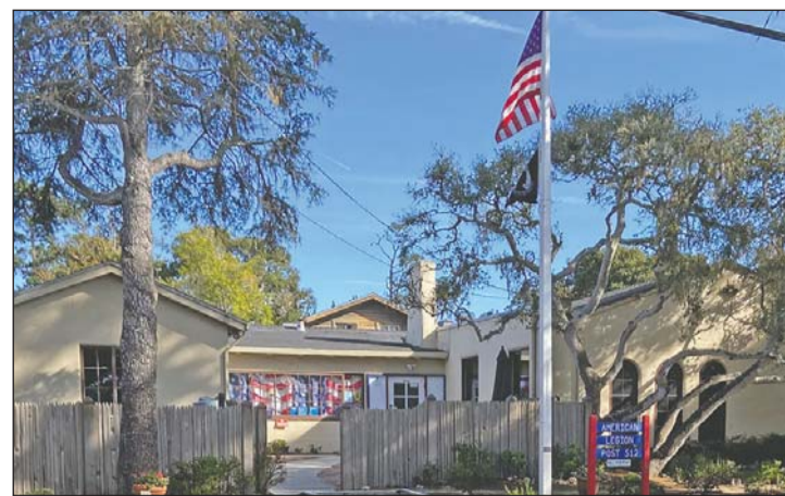
A current image of American Legion Post No. 512, which has been housed on the east side of Dolores just south of Eighth since it was formed in 1934.
