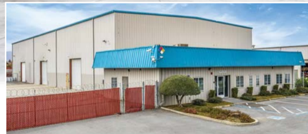
1650 Lana Way, Hollister -Main Warehouse is 15,100 sq ft
