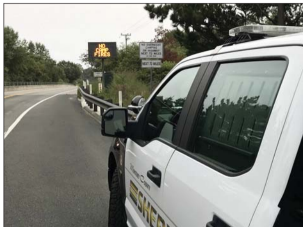
Near Carmel Bridge along Highway 1, signs alert motorists to camping and campfire restrictions. Similar signs will be posted along Nacimiento-Fergusson Road to deter illegal activity.
