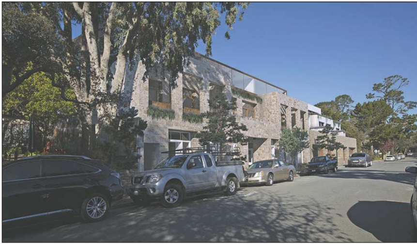
This rendering shows architect Erik Dyar's vision for Del Dono Court 2, but with the project stalled out and the whole thing for sale, who knows whether it will ever be built?
