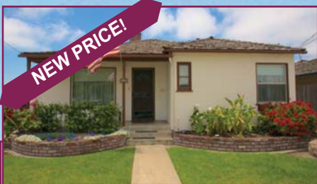
PLENTY OF ROOM in South Salinas 42 Nacional Street, Salinas Open Sunday 1:00 - 3:00 Great location • large bonus room/family room/storage • 3 bed/3 bath $549,900
