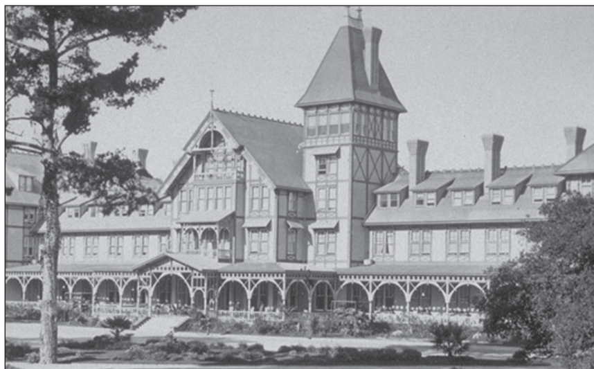
The original Hotel Del Monte, built by the Big Four’s Pacific Improvement Co. as the Southern Pacific Railroad completed its branch line to Monterey in 1880. A young S.F.B. Morse was put in charge of most the railroad’s real estate holdings, including the hotel, in 1915.
