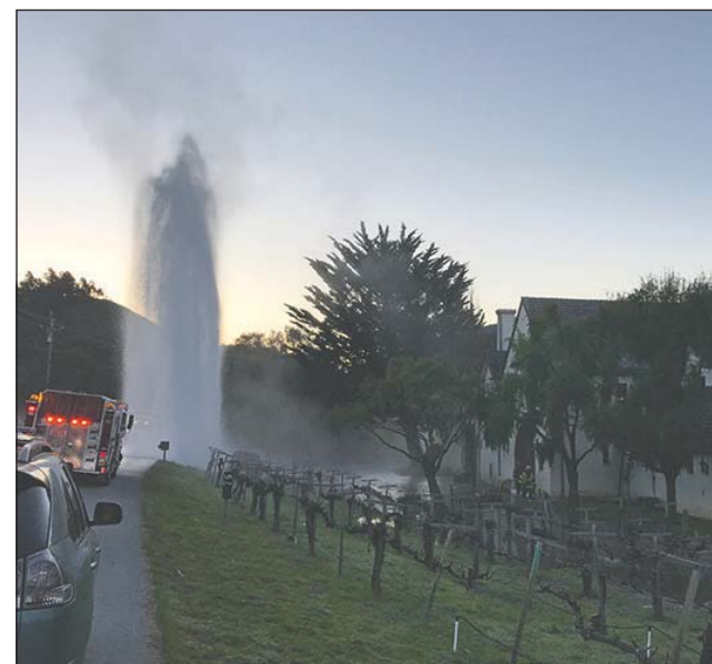
A truck hit a fire hydrant near Folktales Winery Feb. 19, creating a spectacular 50-foot geyser, which continued for at least a half-hour, according to onlookers. "Due to the amount of water at the site, it was challenging for our operators to find the valve and close it off," Cal Am spokeswoman Catherine Stedman said. The amount of water lost is unknown, but since the geyser happened in Carmel Valley, the water just flowed back into the Carmel River, which is where it came from.
