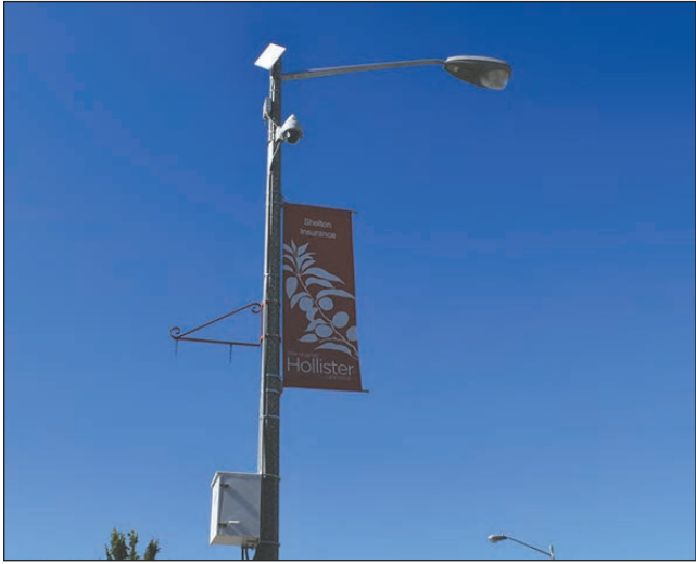
SurveillanceGrid, the company hired to install and maintain surveillance cameras that will log the license plates of every car driving into and out of town, received a national award for a similar project in Hollister.
