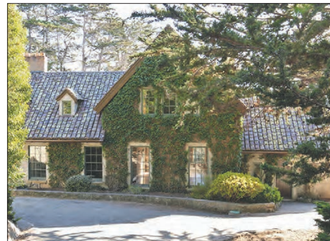
Will someone move into the aging Flanders Mansion and restore it? The city council is leaning toward that scenario as the best option.
