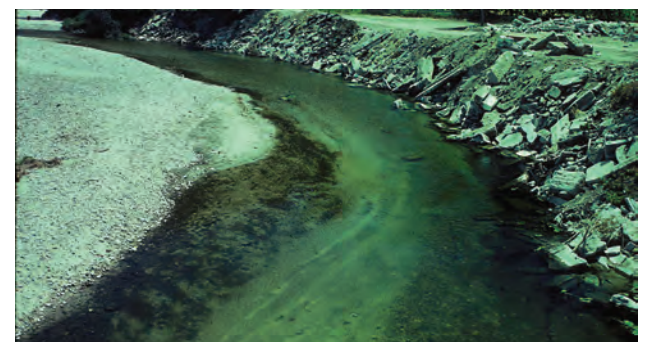
Pictured above are the banks of the Carmel River near the Schulte Bridge in Carmel Valley following years of over-pumping. Circ. early 1990's
