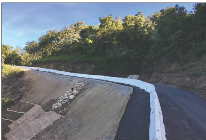
A one-lane temporary road was opened on Cachagua Grade last spring so locals could use the road, but now it's closed again while Granite Construction works on a permanent fix.
