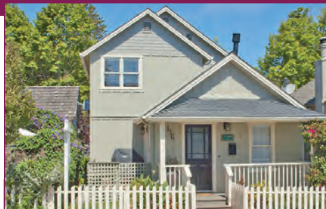
REMODEL IN THE RETREAT 136 19th St, Pacific Grove
