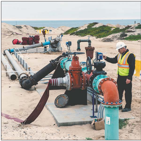
A Cal Am engineer checking a desal plant test well located at a sand mine in the Marina Dunes that’s set to close.
