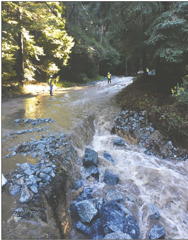
PHOTOS/COURTESY CALTRANS, CHRIS COUNTS
