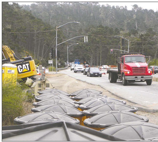
Construction equipment and collision barriers (left) line Highway 68 near its junction with Highway 1 as workers start building the much anticipated roundabout (right) which is expected to smooth traffic by eliminating the stoplight and all left turns at the busy intersection.
