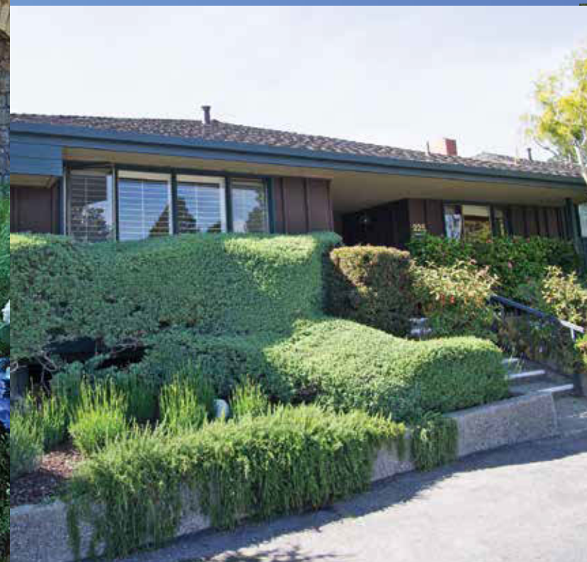
225 Del Mesa Carmel | Pristine Remodel On Coveted Lawn Bowling Green | $785,000
