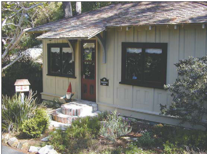
The aptly-named Door House sits proudly on its third lot, this one on Pescadero Road. It's just one example of Carmelites' predilection to move buildings for preservation — or for profit.
