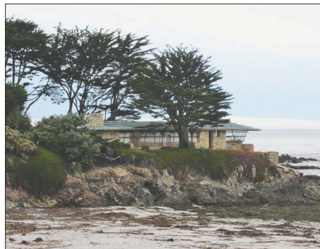
A new seawall will protect the historic Frank Lloyd Wright house from being ravaged by waves, and it's been designed to blend in with the natural rock face above the beach.
