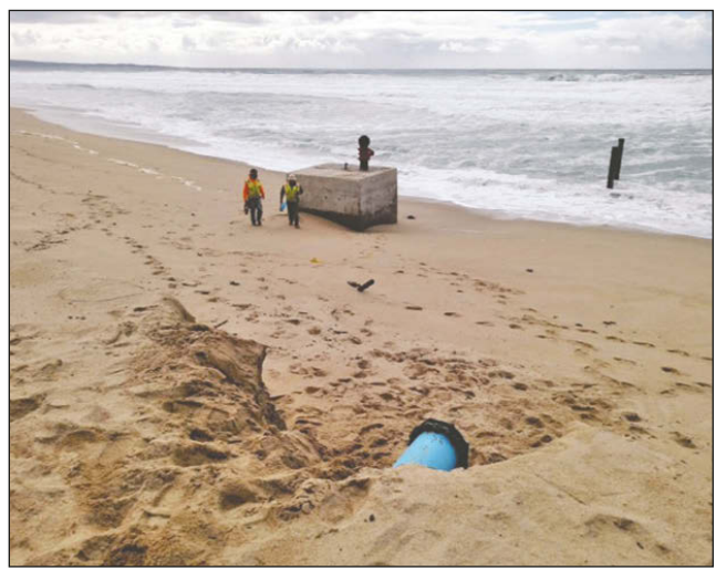
The pipe that connected Cal Am's desalination test well to a concrete vault was exposed by beach erosion during recent storms (top) and then became detached Monday (right). Though repairing the pipe would be easy, it may take months for the Cal Am to get approval from the coastal commission to fix it.
