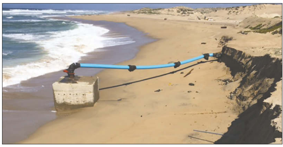
The pipe that connected Cal Am's desalination test well to a concrete vault was exposed by beach erosion during recent storms (top) and then became detached Monday (right). Though repairing the pipe would be easy, it may take months for the Cal Am to get approval from the coastal commission to fix it.
