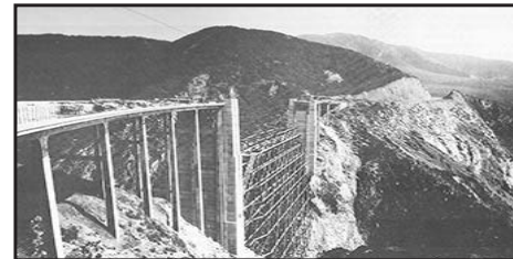
Construction of Bixby Bridge
