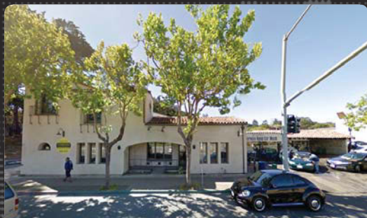
Myrick - El Estero Building 590 Fremont Street Monterey, CA
