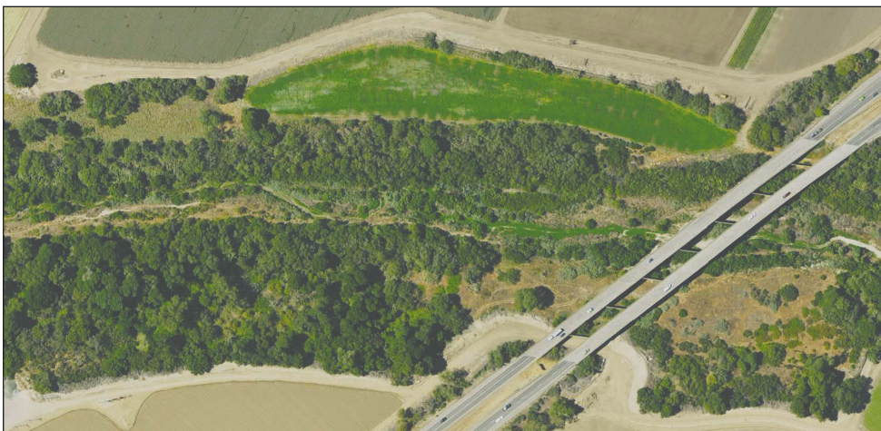
As shown in this aerial of the Highway 68 crossing, the Salinas River channel is choked with trees and shrubs, and presents a serious flood danger if heavy rains come this winter, farmers say.
