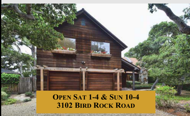
Pebble Beach ~ Spacious home offers excellent floorplan with vaulted ceilings & 3 fireplaces. 5 Bedrooms ~ 4 Baths $1,375,000
