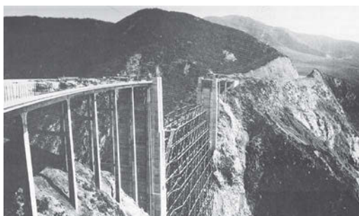
In 1931 M.J. Murphy was one of the sub-contractors involved in the construction of the Bixby Bridge. Murphy truck drivers made the dangerous trip many times supplying the materials needed.
