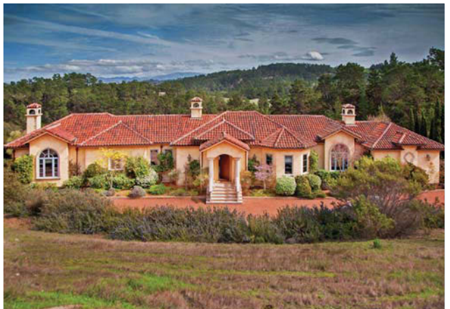
7422 Alturas Court, Monterra 4 Beds, 4+ Baths $3,495,000
