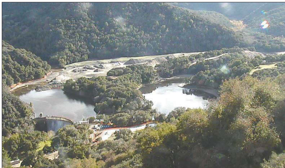
A Cal Am web cam this week showed water spilling over the San Clemente Dam (lower left). By the end of next year, if all goes according to schedule, the dam will be removed.
