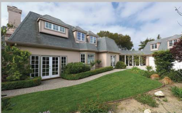
Carmel ~ Mathams designed home . . . French Provincial architecture with a modern day floor plan 4 Bedrooms ~ 5 Baths $2,395,000
