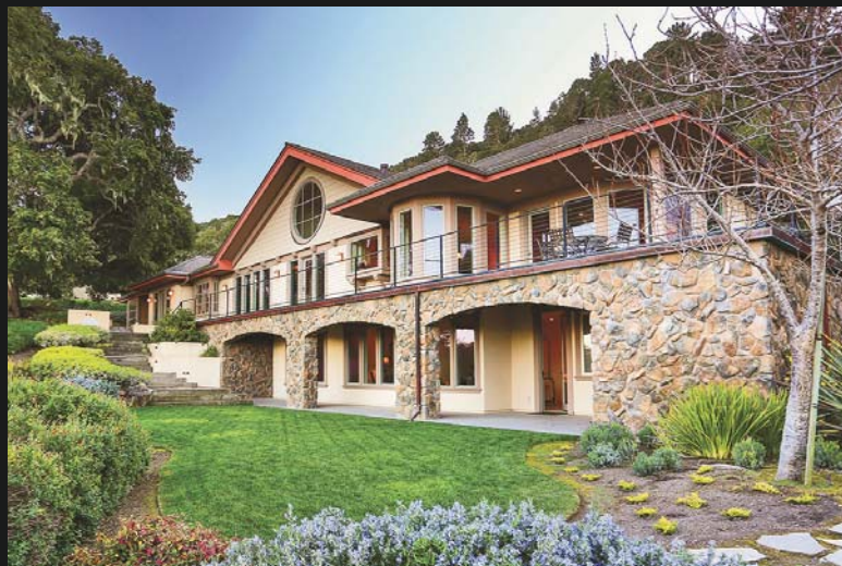
GATED DRIVEWAY • 2002 CONSTRUCTION
