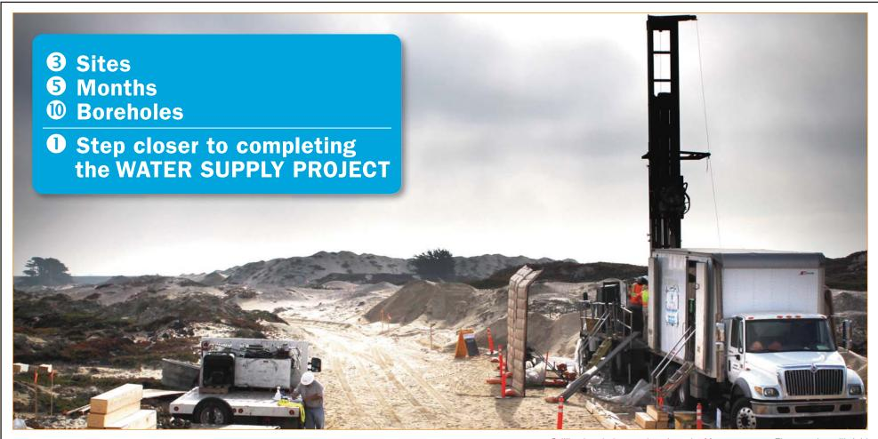
Drilling borehole samples along the Monterey coast. The samples will yield critical data needed for environmental impact and technical review.
