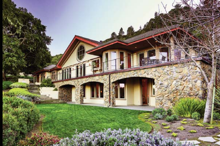
GATED DRIVEWAY • 2002 CONSTRUCTION
