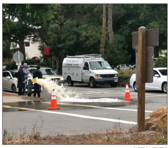
Workers for Cal Am let a hydrant run at the corner of Juniper and Ocean Friday morning to help flush discolored water from the mains.
