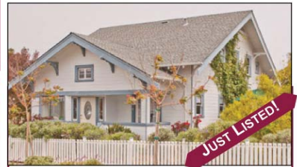
GRACIOUS CRAFTSMAN 440 Junipero Ave, Pacific Grove Open Saturday 2:00 - 4:00 Authentic period details • 5bds/3ba • peek of Bay • finished basement $895,000
