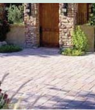
Paving and stonework
