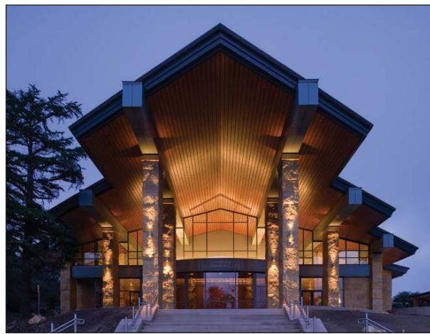
The performing arts center at Carmel High School earned the school district and its architect, Peter Kasavan, a statewide Award of Excellence for its design.
