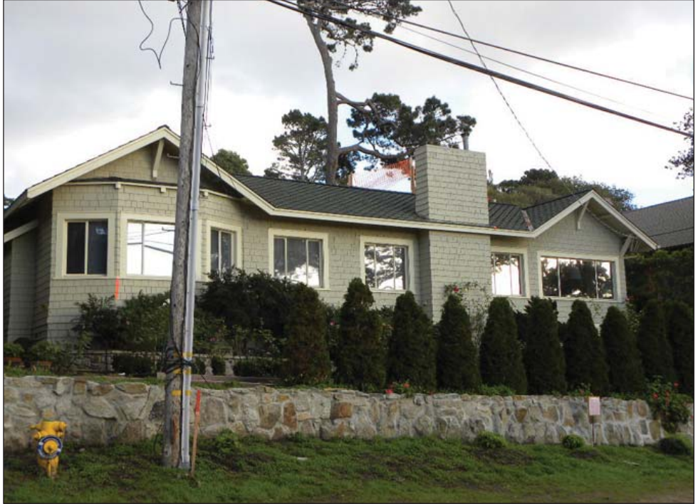
This home at Carmelo and Ocean is slated for demolition, since it's full of mold, but the planning commission has to OK its replacement, first.
