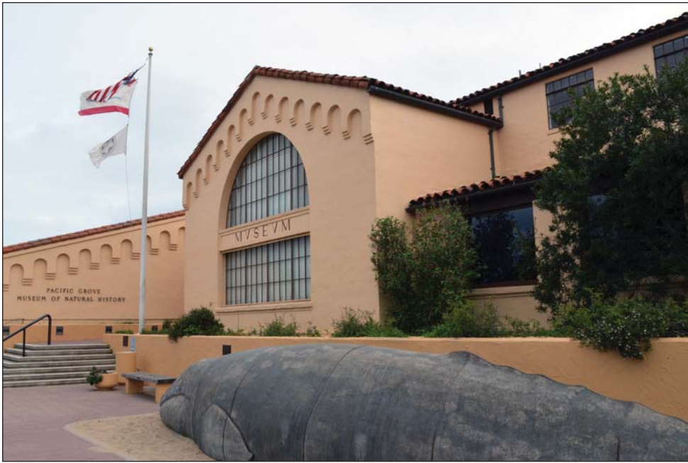
The Pacific Grove Museum of Natural History's older wing (right side of photo) was built in 1932, and the museum's director is expressing concern about the safety of its foundation.
