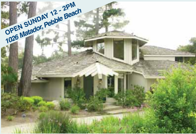
Entertainer's Villa. Vaulted ceilings. Open floor plan. 8-sided rooms. Seller finance. 2,996 sq. ft. $1,200,000 www.PebbleBeachVilla.com
