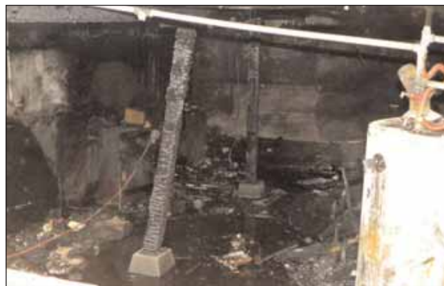
PHOTO/COURTESY MONTEREY FIRE
