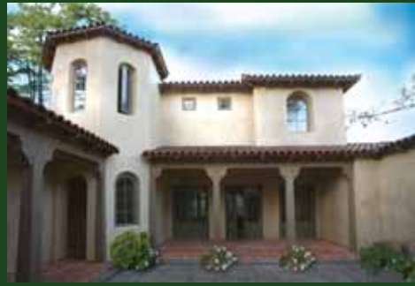
New Construction - Traditional Spanish Revival $3,695,000 www.2971Cormorant.com
