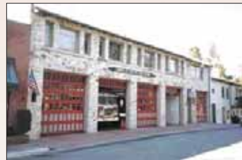
CARMEL FIRE STATION RETROFIT
