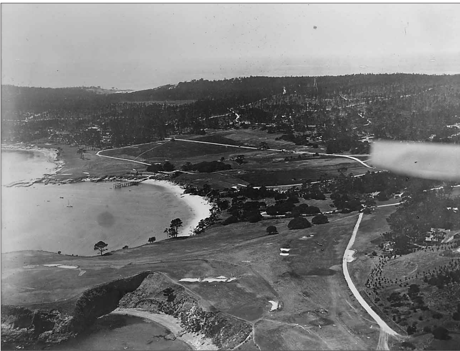
An aerial view of the Pebble Beach Golf Links in 1919, the year the course opened.
