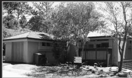
2 SE of 2nd & Carpenter
