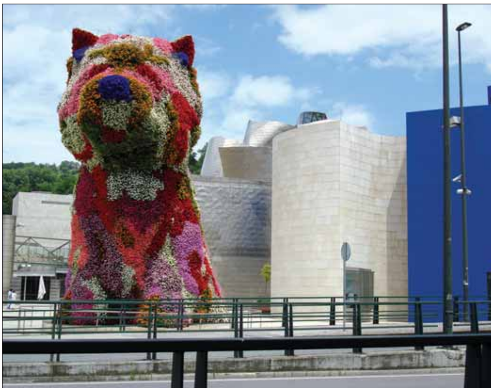
The Guggenheim Museum in Bilbao, Spain, is a cousin to Los Angeles' Disney Concert Hall. Both were designed by Frank Gehry ... but the Los Angeles version doesn't come with a giant flowered dog.
