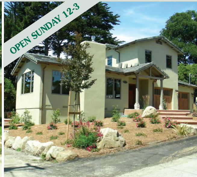
25238 HATTON RD TOTAL REMODEL
