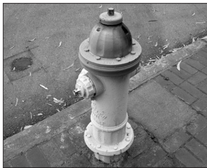
If this were a color photo, you could tell how much water the hydrant is supposed to deliver.
