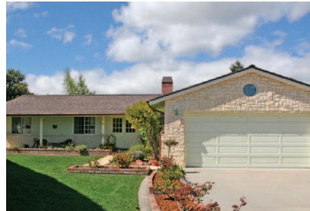
CORRAL DE TIERRA Sunny & Quiet: Remodeled 4BR/2BA home is located on a quiet cul-de-sac with easy access to highway. Kitchen boasts handcrafted pine cabinets & granite counters. Saltillo tile floors. Stone patio. $1,095,000. 831.624.0136
