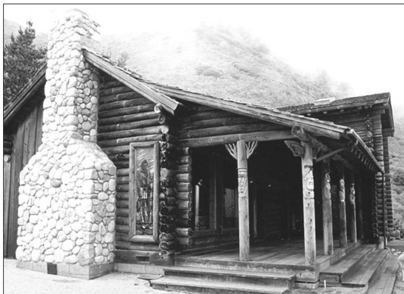
Behind the ridge at Brazil Ranch, a collection of historic buildings is being used for commercial functions, upsetting some residents of a Big Sur residents.
