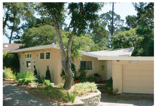
MONTEREY Showered with Light: With 1,569 sq. ft. of living space & over 1,000 sq. ft. of outdoor decking, enjoy the view of the verdant green canyon. Huge windows replace walls & recently remodeled kitchen. $869,000. 831.646.2120
