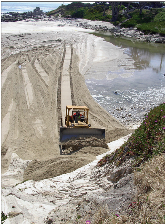
In an effort to fortify Scenic Road and a landmark cypress tree, a Monterey County Public Works bulldozer operator piles up sand against the eroding bluffs.
